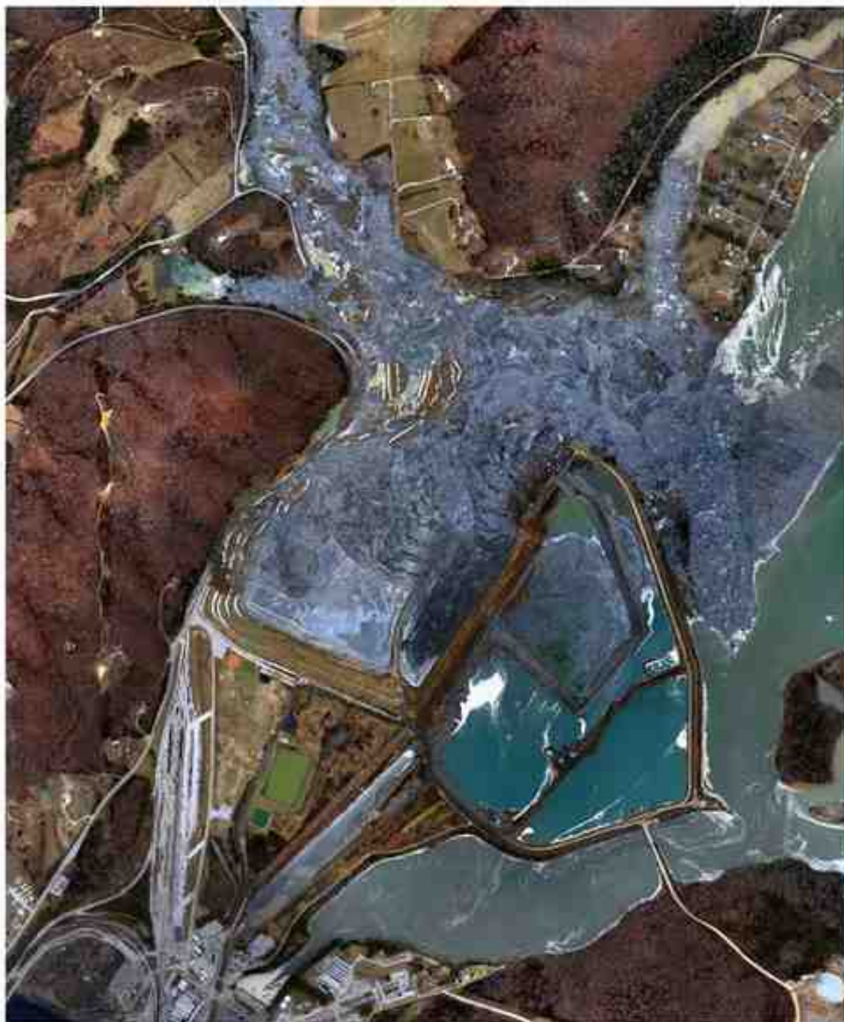
Aerial Image Of Kingston Ash Slide 12/23/08
